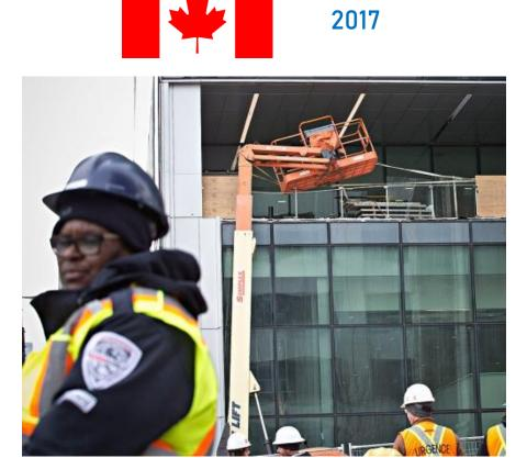
The MEWP was traveling on a granite surface when it rolled over a wooden panel that covered a hatch on the ground. "*There was snow on the ground. It is very likely that the worker did not see the wood panel because of this snow*" The MEWP then tipped over against the building under construction
